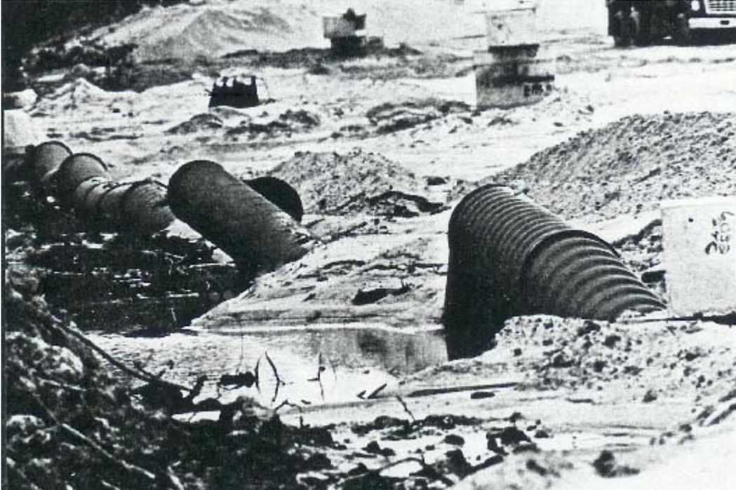
*PVC Profile Gravity Sewer Pipe floated after installation due to groundwater conditions.*
