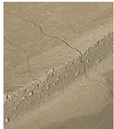
The 0.04-inch crack shown is less than half the crack width of 0.10-inch accepted by Caltrans and AASHTO.
