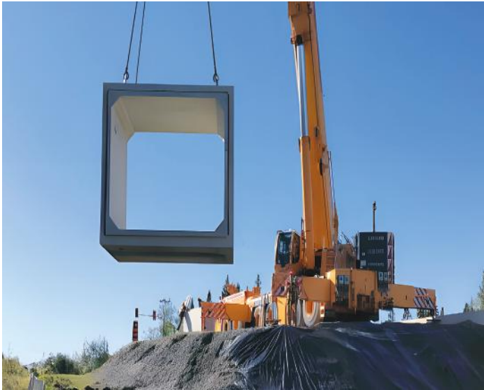
Box Culverts with Spans Greater Than 3000mm
